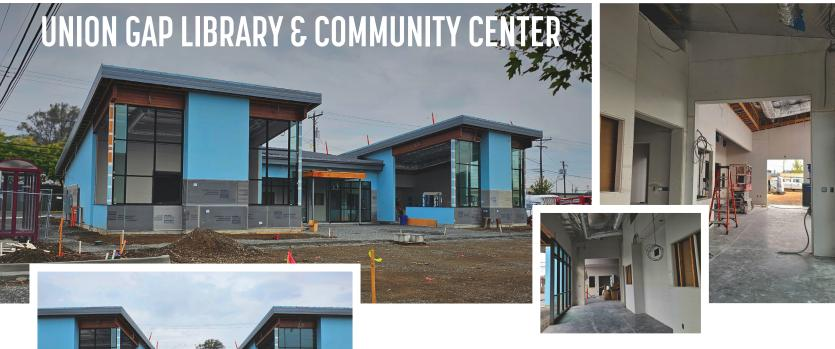
The new **Union Gap Library and Community Center** is moving right along! The walls are up and plumbing, mechanical, and electrical rough-in are in full swing. The roof was installed, and things will be really starting to take shape. As construction continues to progress, we expect to have the project complete this coming spring!
