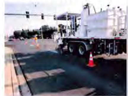
Valley Mall Boulevard Resurfacing Phase 2
