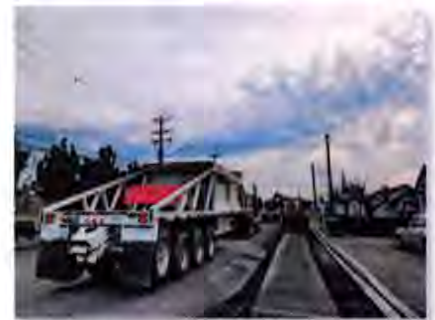
West Ahtanum Road Resurfacing
