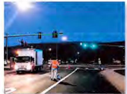
Longfibre Road Resurfacing
