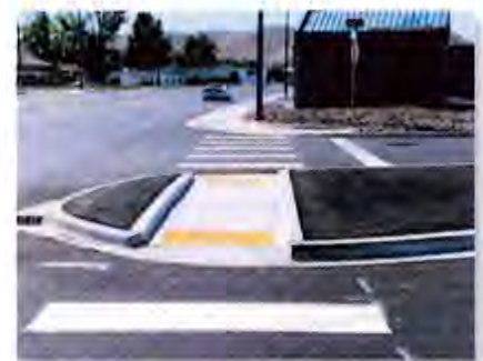
Main Street Reconstruction Phase 1
