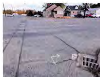
Current conditions along Main Street
